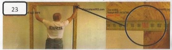
Prepare the two screen tracks: (V) – height 36 mm and (U) – height 25 mm (figure 24), align the brush strips at the ends (figure 25), and determine the position of the cut =
